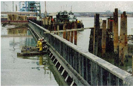
Wilmington Harbor Sheet Pile - View behind pile as project nears completion.
